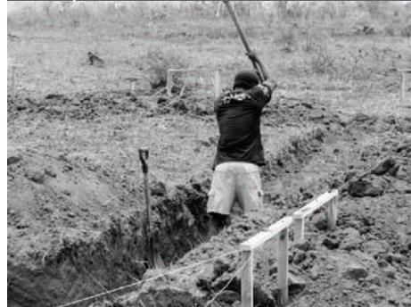
September 2010: Workers begin hand-digging the foundation for the laboratory building.
